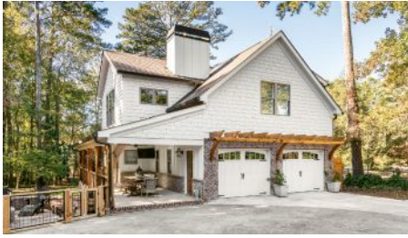
Residential Detached Structure Ranney Blair Home Renovations Roswell, Georgia
